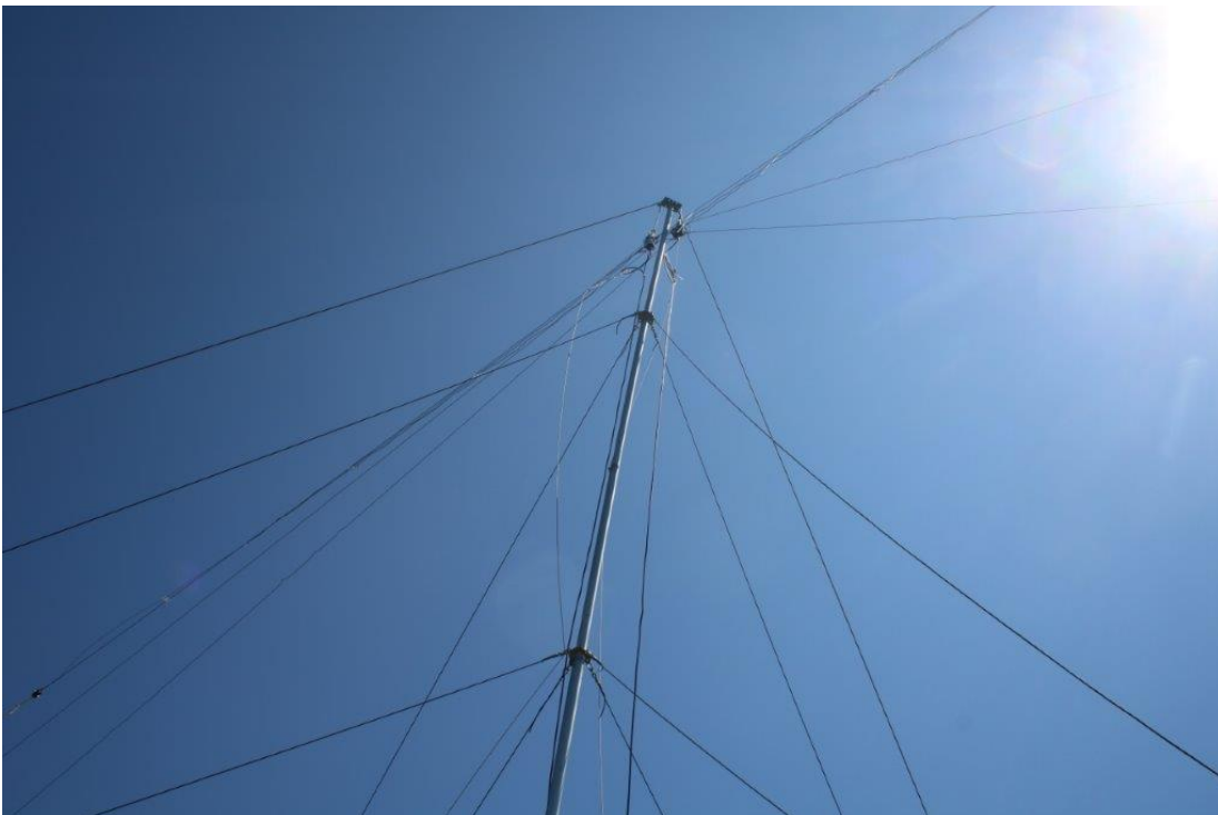
VIEW UP THE MAST SUPPORTING THE FAN DIPOLES (NOTE BLUE SKY & SUNSHINE!!)
