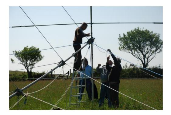
But there is a better way! It involves the use of a device usually called a tilt plate, which allows both mast and antenna to lie flat at ground level, enabling the antenna and feeder to be connected to the mast in safety at a comfortable height, and then tilt the mast up to vertical while keeping the antenna horizontal.
