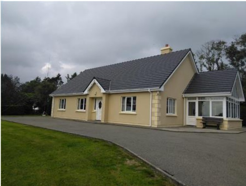
HOUSE – ONE MILE NORTH OF BANTRY BAY
