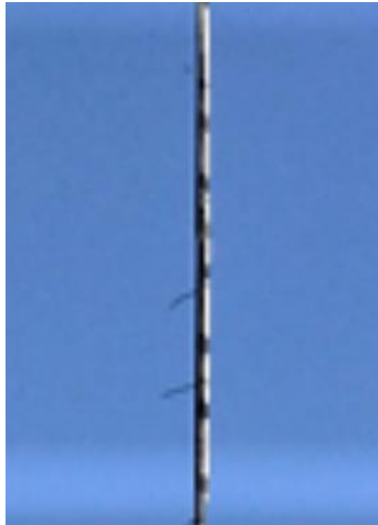
FIBREGLASS ROACH POLE REPAIRED WITH PVC CONDUIT
