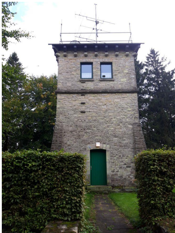
An older stone tower with various antennas on and around it
